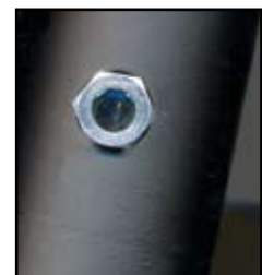
This sight gauge shows the color of the silica gel. When the gel turns from blue to pink, it is time to change the desiccant.
