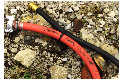
Zip tie or strap hoses together
