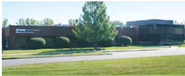
Fluid Control Division Headquarters, New Britain, CT.
