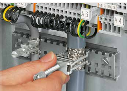
Securing an additional shield clamping saddle.
