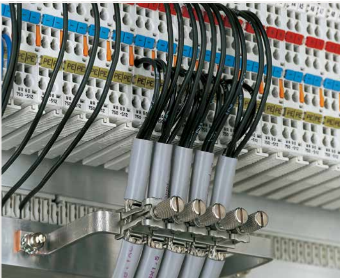
U-shaped (10 x 3) mm copper busbar
