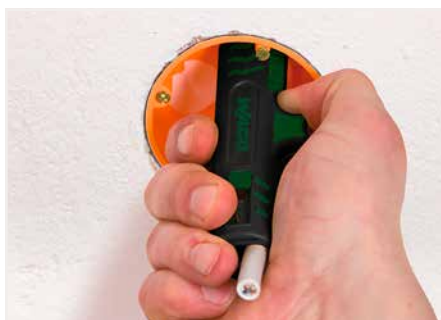
Stripping a cable sheath.
